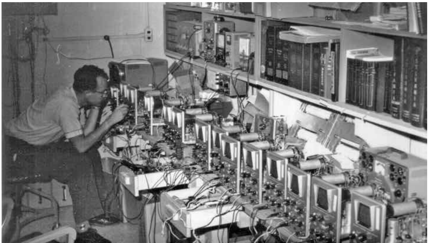
Figure 3: A lineup of 14 IO-21 Oscilloscopes undergoing evaluation by a technician at the Heathkit factory. It was customary to have Heath employees build new kits for evaluation. Construction experience data was given to the manual department, and the completed kits were evaluated by technicians for performance. Photo from Gene Fiebich via Chuck Penson.
